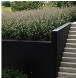
Concrete wall Rendered and painted in black
