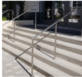
Metal Flatbar Stair Handrails
